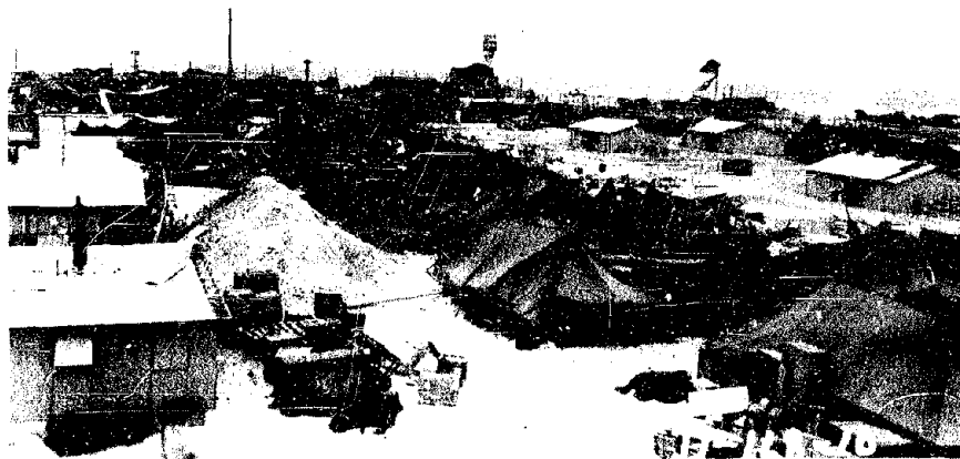
Fig. 3.5 Camp and Warehouse Area, Tare Island Postshot, 14-3/4 Miles from GZ
